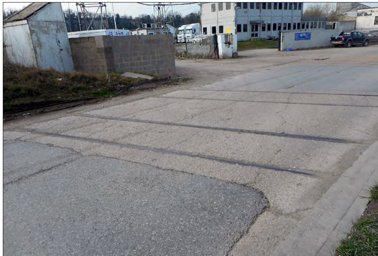
Plate 7) Tramline within the Site across Manor Way
