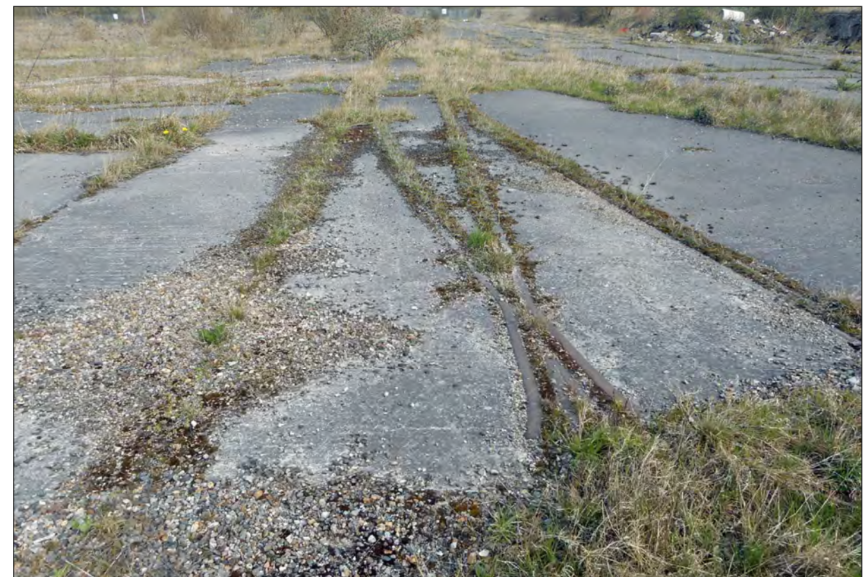
Plate 8) Section of tramline within the Site (WA790)
