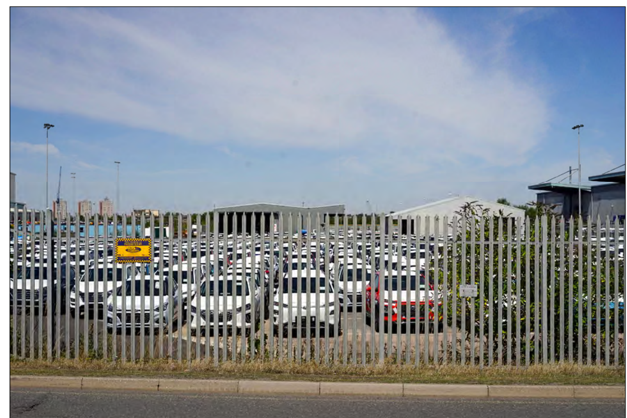
Plate 22) View of the central part of the Essex Project Site looking north
