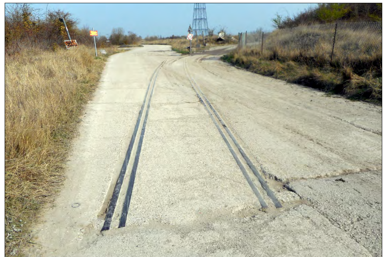
Plate 10) Section of tramline within the Site (WA790)
