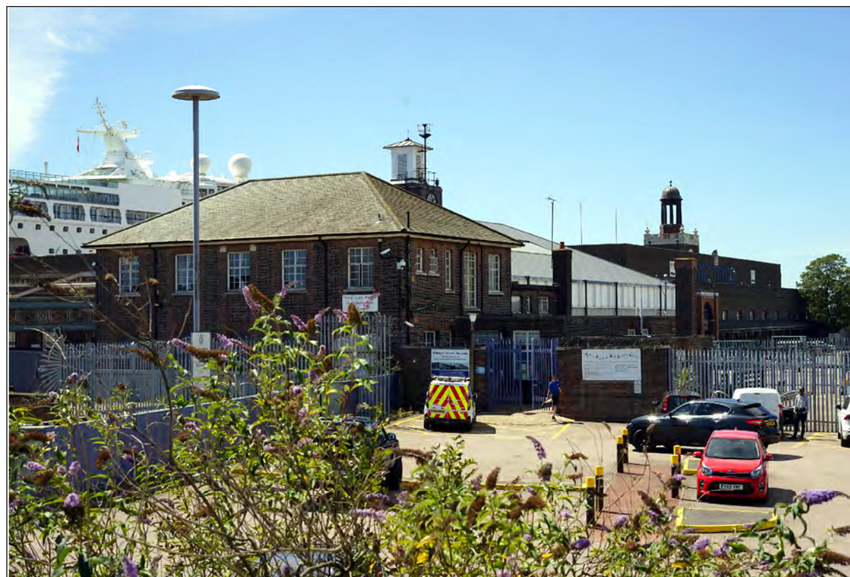
Plate 17) View of Riverside Station building looking south west
