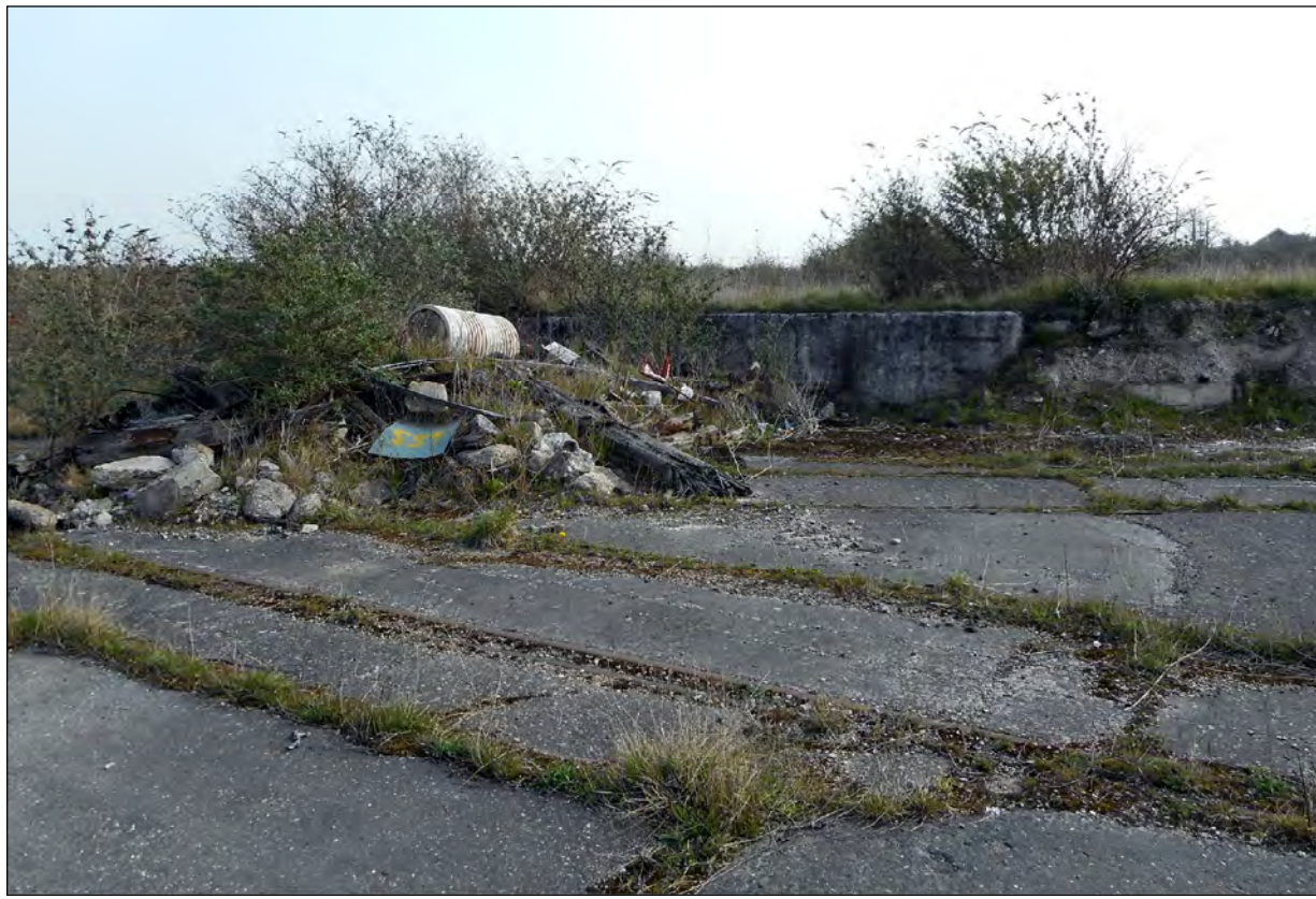
Plate 9) Section of tramline within the Site (WA790)
